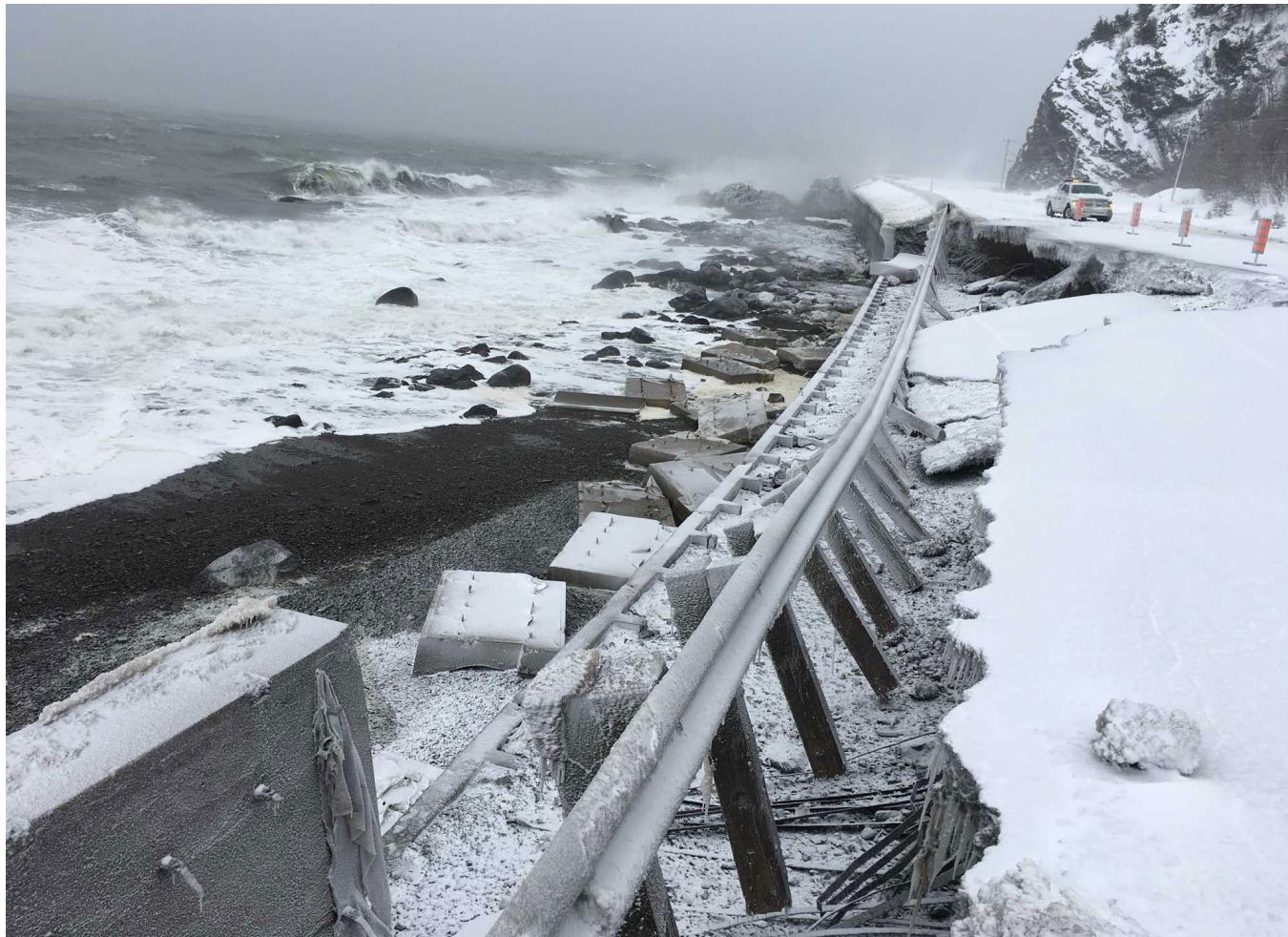
Figure 2.8: Sections of Route 132 washed away in La Martre, Gaspé. Source: Sûreté du Québec, 2016.
