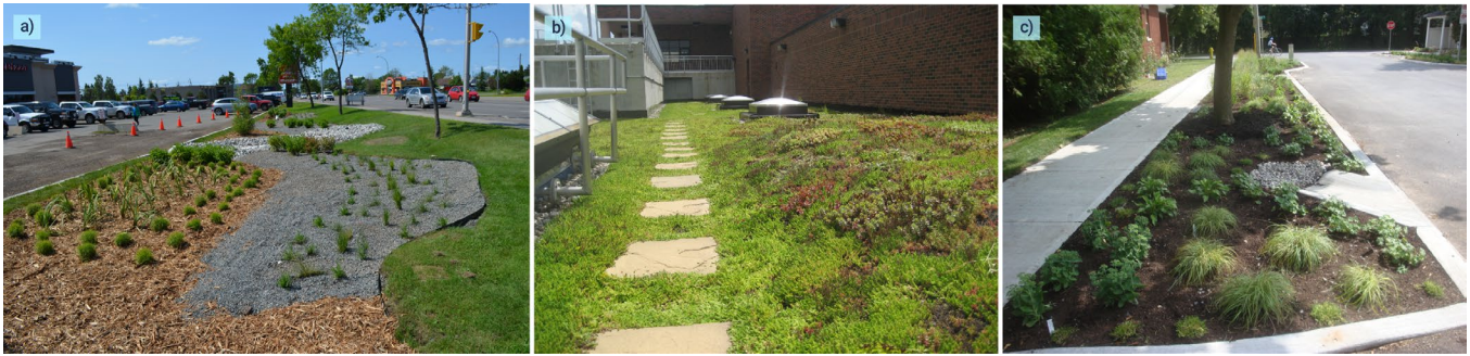
Figure 3.13: Three examples of low-impact development projects. a) Memorial Avenue biofiltration low-impact development in Thunder Bay. b) Green roof low-impact development on the Lou Romano Water Reclamation Plant in Windsor. c) Alwington Avenue bioswale project in Kingston. Sources: a) City of Thunder Bay, 2015; b) Courtesy of the City of Windsor; c) Courtesy of the City of Kingston.
