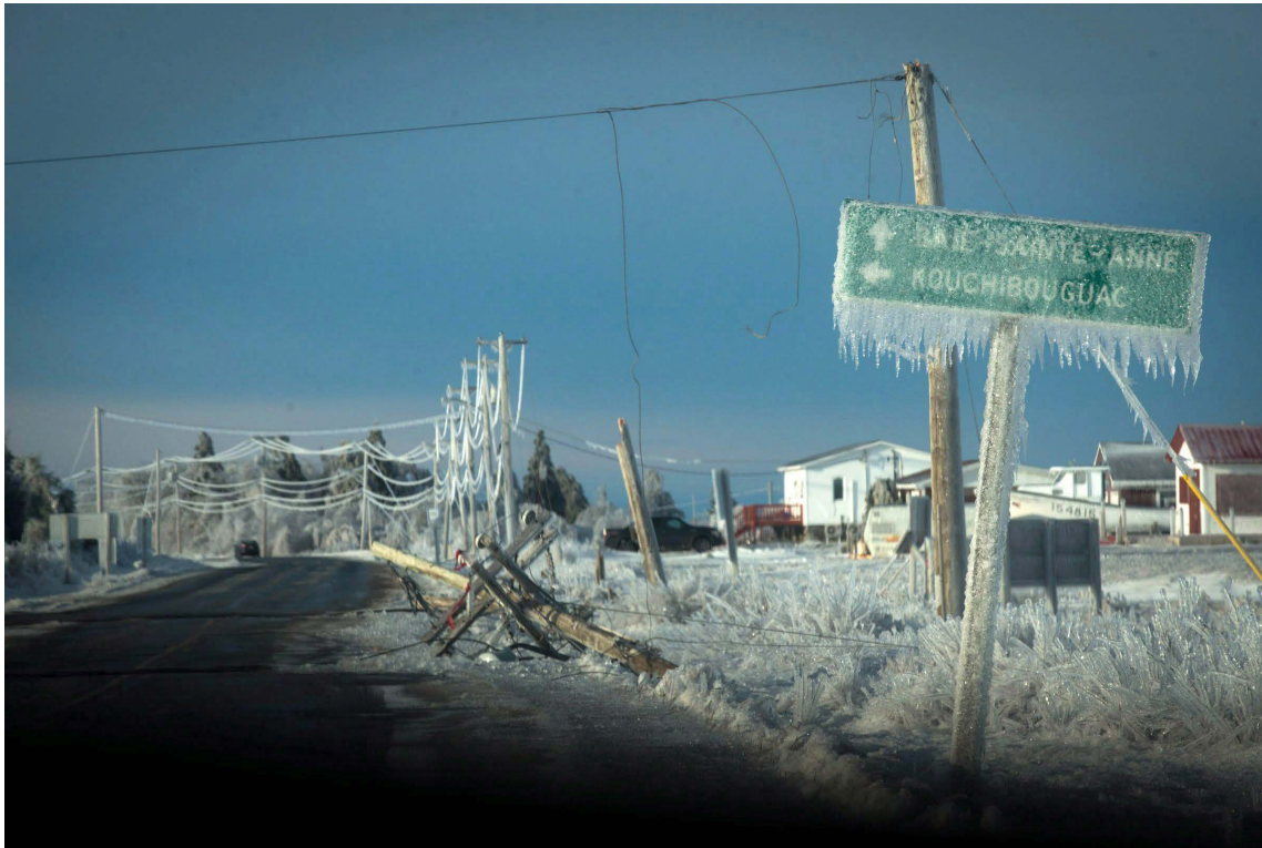
Figure 1.9: Damage caused by the 2017 ice storm in the Acadian Peninsula. Source: The Canadian Press/Diane Doiron
