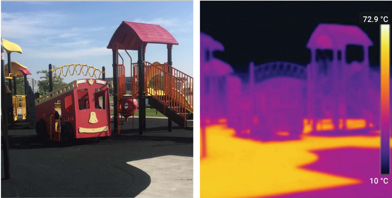
Figure 2.10: Thermal imaging of Windsor's Captain John Wilson park shows that the temperature of the dark rubber mat under the play structure (yellow area) is 69.0°C. Photos courtesy of the City of Windsor.
